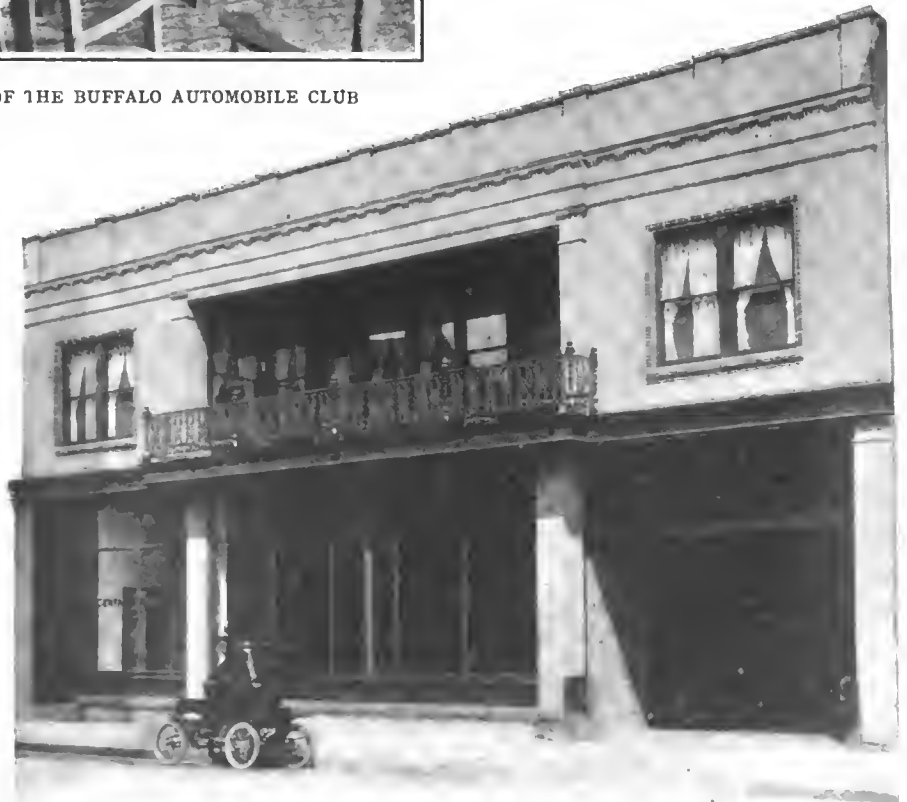
BUILDING ON FRANKLIN STREET, BUFFALO, IN WHICH CLUB ROOMS ARE LOCATED.
